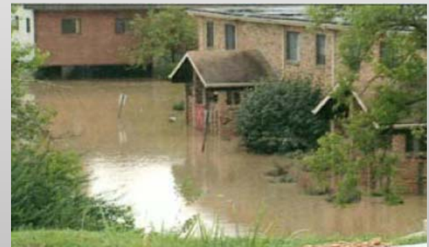
Flooding in Brentwood, Mo. (Photo credit: Scott Thomas/KMOV)
