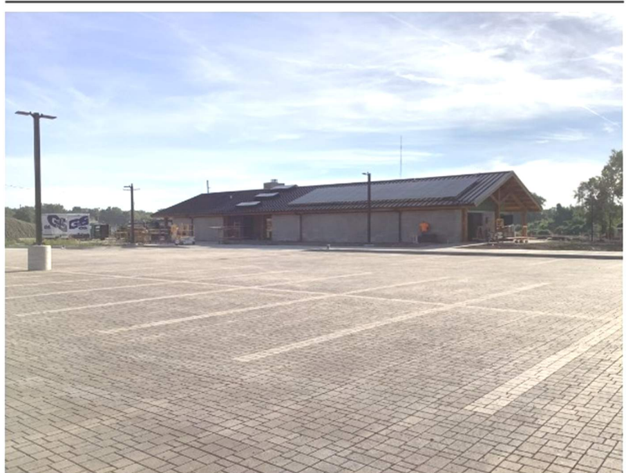
Comfort Station (Pavilion) structure as viewed towards the northeast from the permeable paver parking lot.
